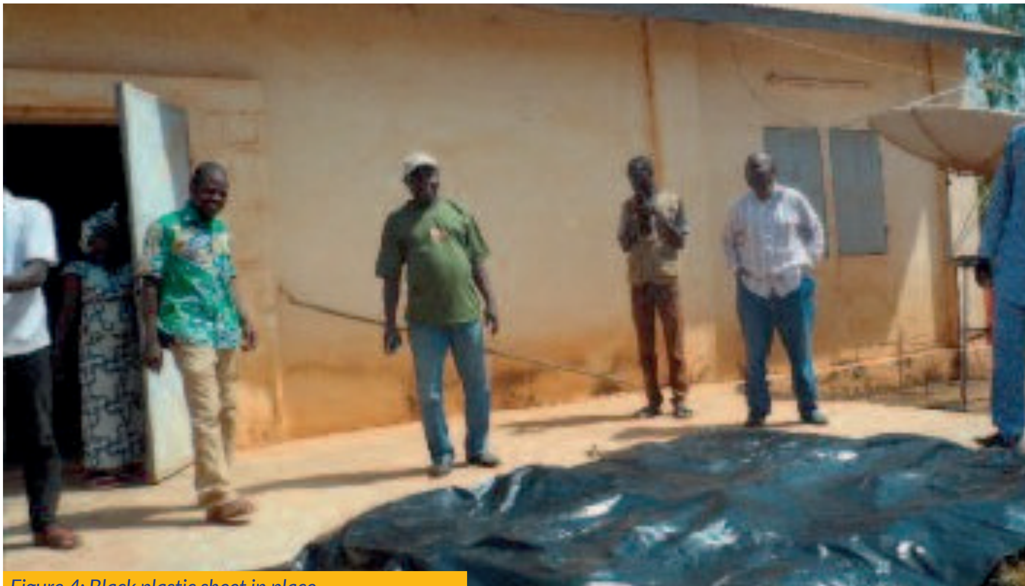
Figure 4: Black plastic sheet in place
